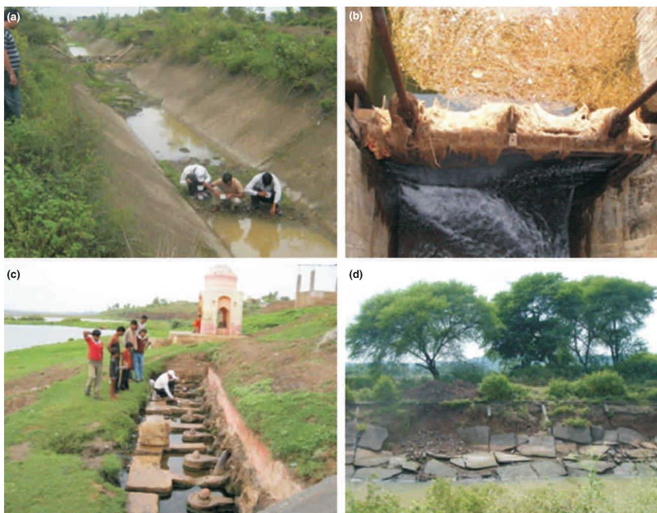
Photographs showing: (a) water stagnation in canal, (b) stagnation at gates, (c) breeding sites at religious places, and (d) broken margins of canal.
