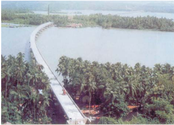
Fig. 114: To lay railway line long bridges had to be constructed over the broad perennial rivers
