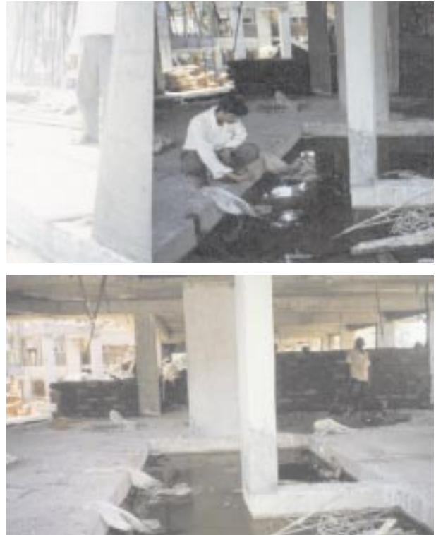
Fig. 123: Curing tanks at construction site in Ward No. 1 and 12 supporting the breeding of An. stephensi during the evidence-based situation analysis survey in Panaji, Goa
