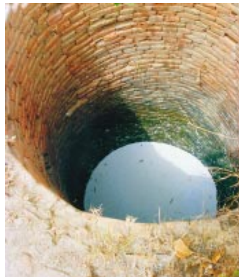
Application of EPS beads in unused wells
